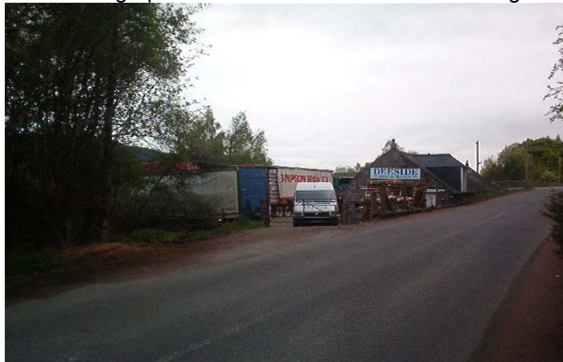
Fig. 2. Site Viewed from the West
